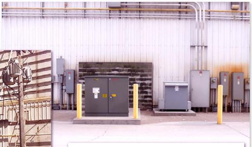
Two overhead 3-phase transformer banks at Yoder Feeds have been replaced by one 3-phase padmount transformer at DeKalb. This set-up reduces outages and congestion, and increases safety.
