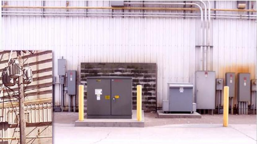
Two overhead 3-phase transformer banks at Yoder Feeds have been replaced by one 3-phase padmount transformer at DeKalb. This set-up reduces outages and congestion, and increases safety.
